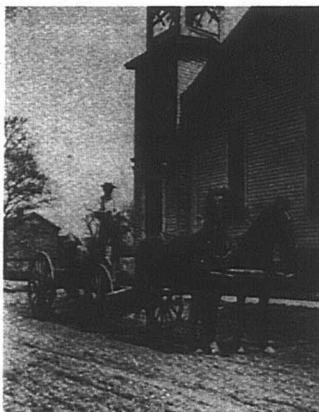
photo courtesy of Luckey Building
