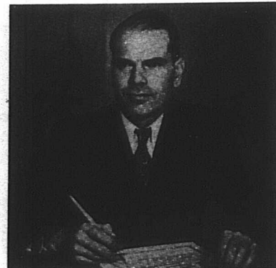
photo courtesy of Luckey Building
