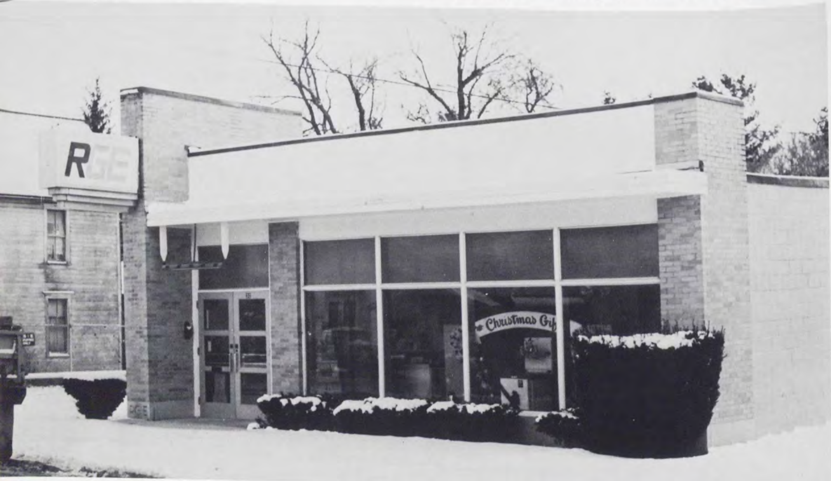
Rochester Gas and Electric
