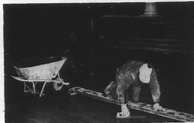
Workmen even the gravel base and smooth the fresh cement of the walk before the Chapel-Auditorium.
