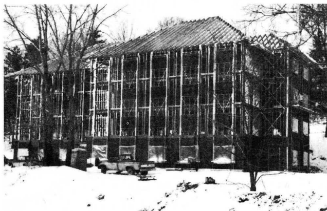
Assembly of its aluminum roof rafters radically alters appearance of the new men's dorm. Enclosure is progressing on schedule despite cold.
