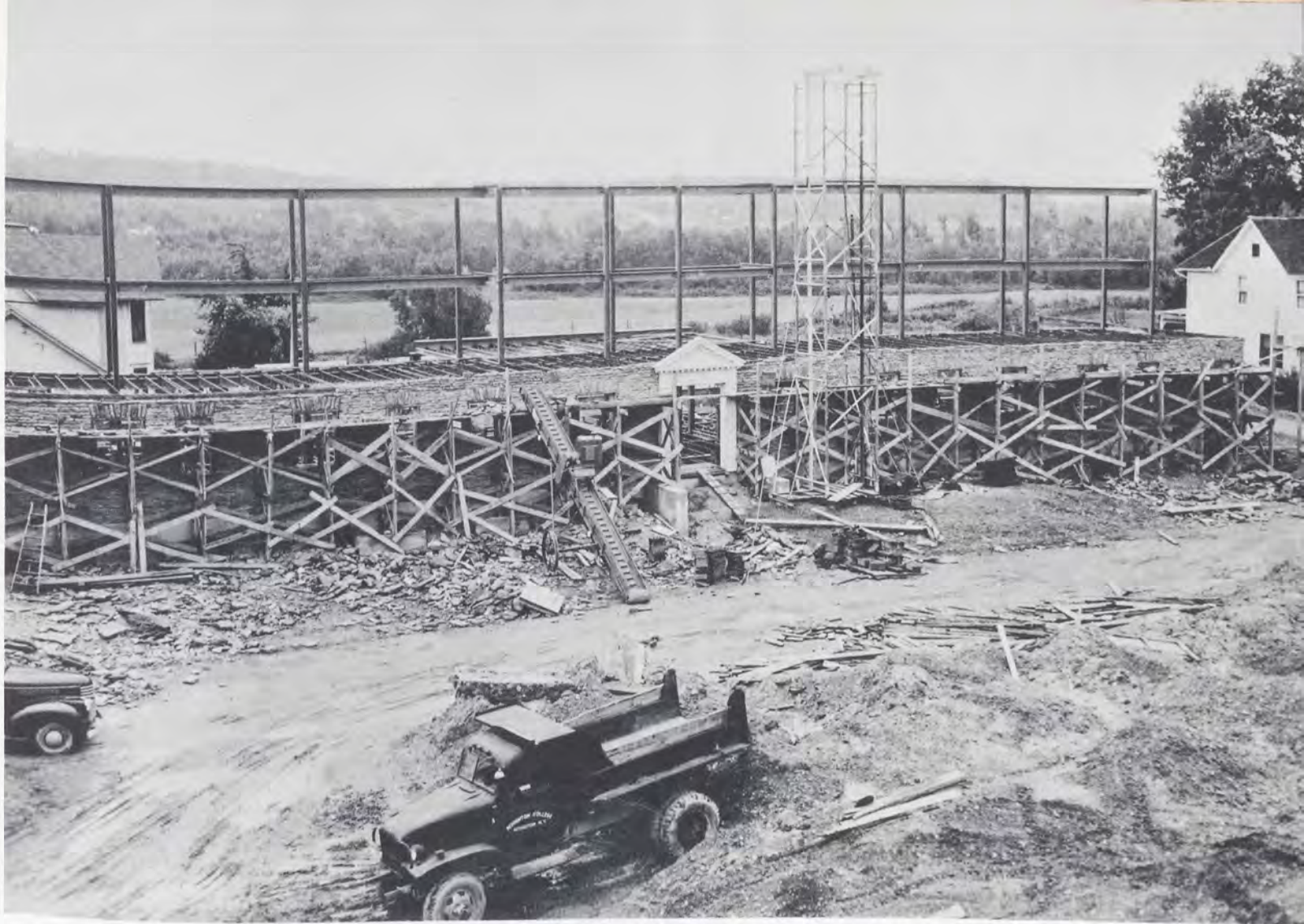
Construction of the main section of East Hall as shown in a 1951 picture— the women's dormitory was the second building to use native stone
