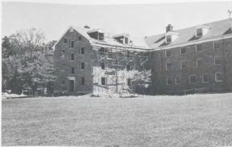
General Contractor of New East Hall Wing
