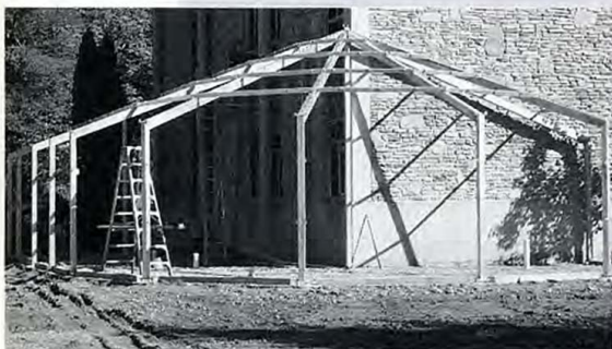
Framing for the Margaret E. Bush Greenhouse completed in May awaits installation of tempered glass panels in June.
