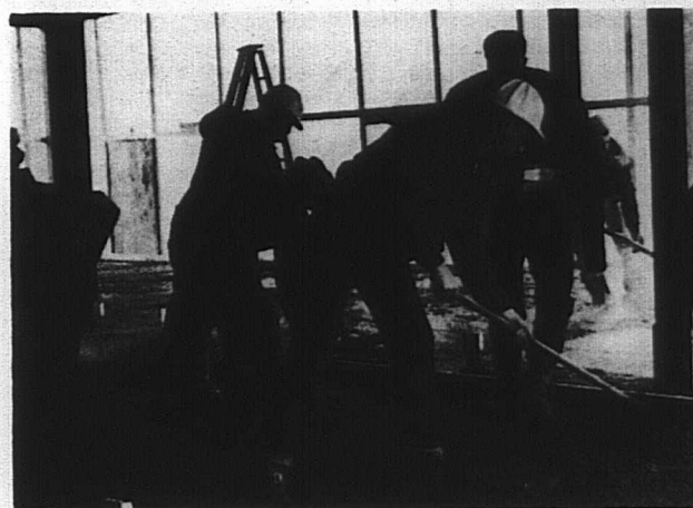
Inside, the steel superstructure, the work continued through the winter and spring of 1969. Artificial heat kept the cement from freezing.
