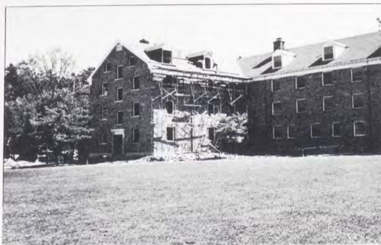
General Contractor of New East Hall Wing
