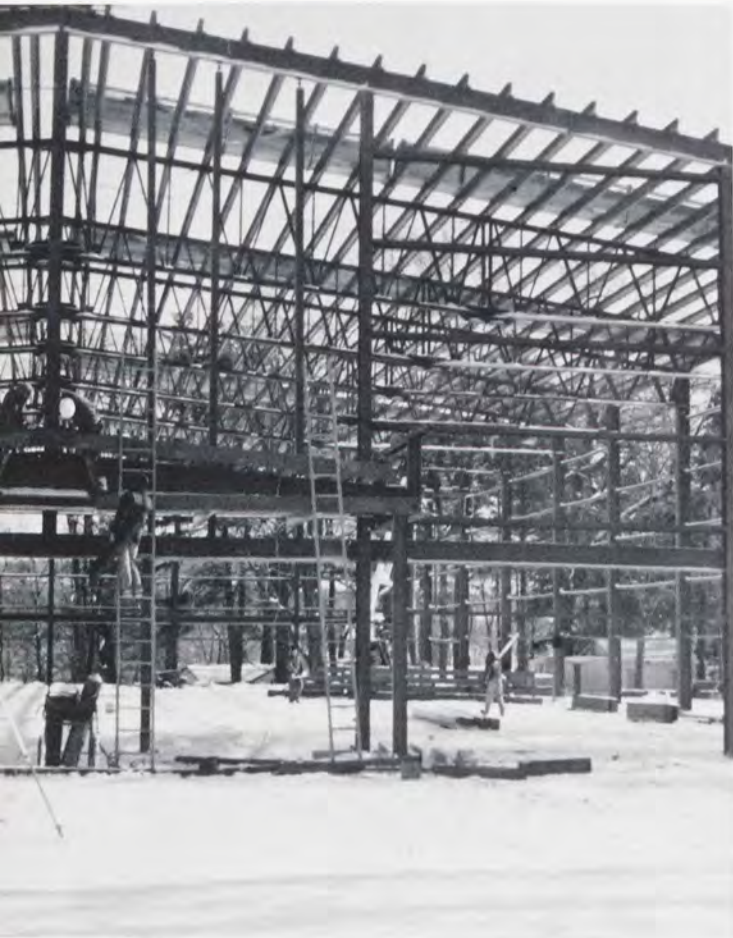
3. girder placing
