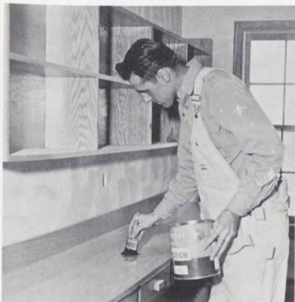
Finishing touches on East Hall wing.
