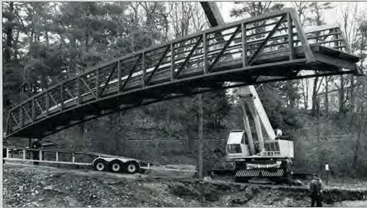
Thanks to gifts by the Classes of 1995 and 1996, a new steel and treated-lumber, arched pedestrian bridge spans Houghton Creek just downstream from Brookside Townhouses. With ramped approaches to facilitate handicapped access, the bridge eliminates need for pedestrians to use the Genesee Street bridge to reach campus. The bridge memorializes four deceased students who would have been members of the giving classes—Chiho Yokota '95, Heather Fronhoffer, Amy Bliss and Michael Smoyer, all of '96.
