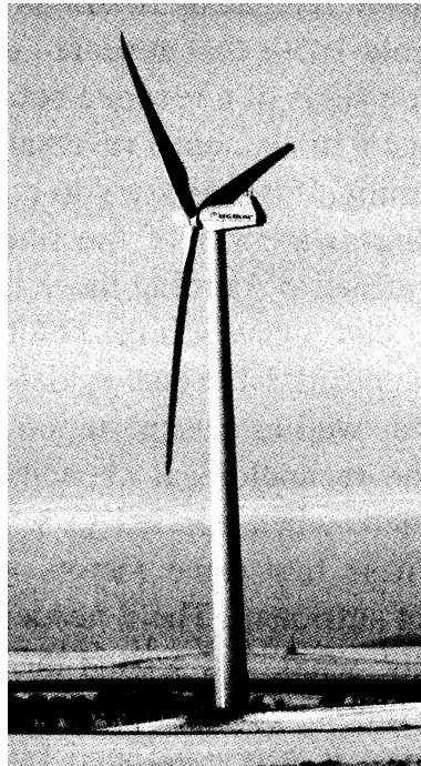
Figure 1. Example of a Modern Wind Turbine. Common three blade upwind turbines have a housing which contains a gearbox, generator, and turbine control systems all mounted on a 100 – 150 ft. tower. Figure taken from Ref [6].
