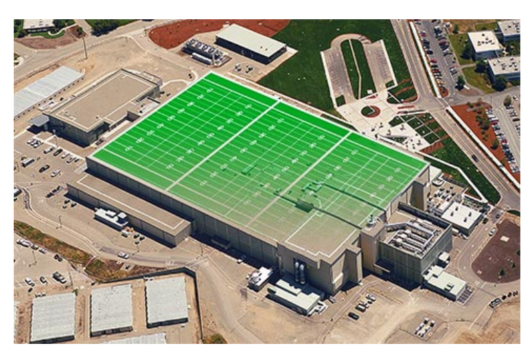
NIF Laser and Target Area Building
